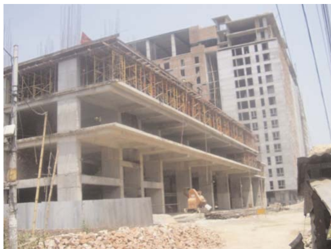
DSE tower, 3rd Floor Construction completed
