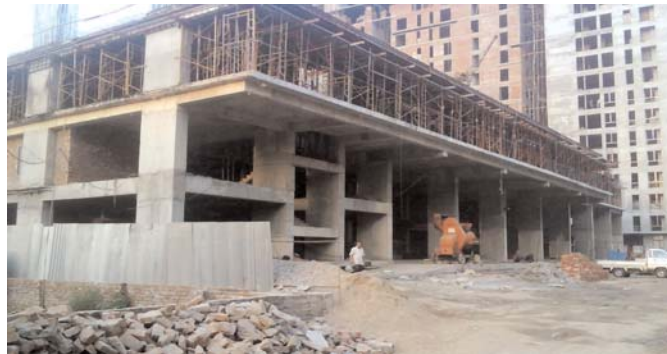
After casting 2nd floor of DSE Tower, Nikunja
