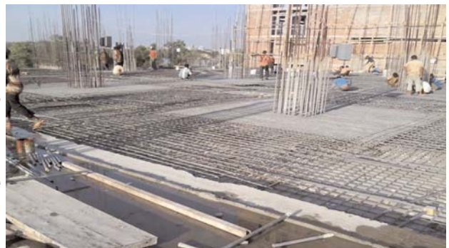
Workers are finally checking their work.
