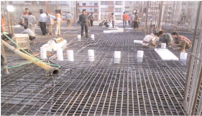
Workers are binding rods before casting under close supervision.
